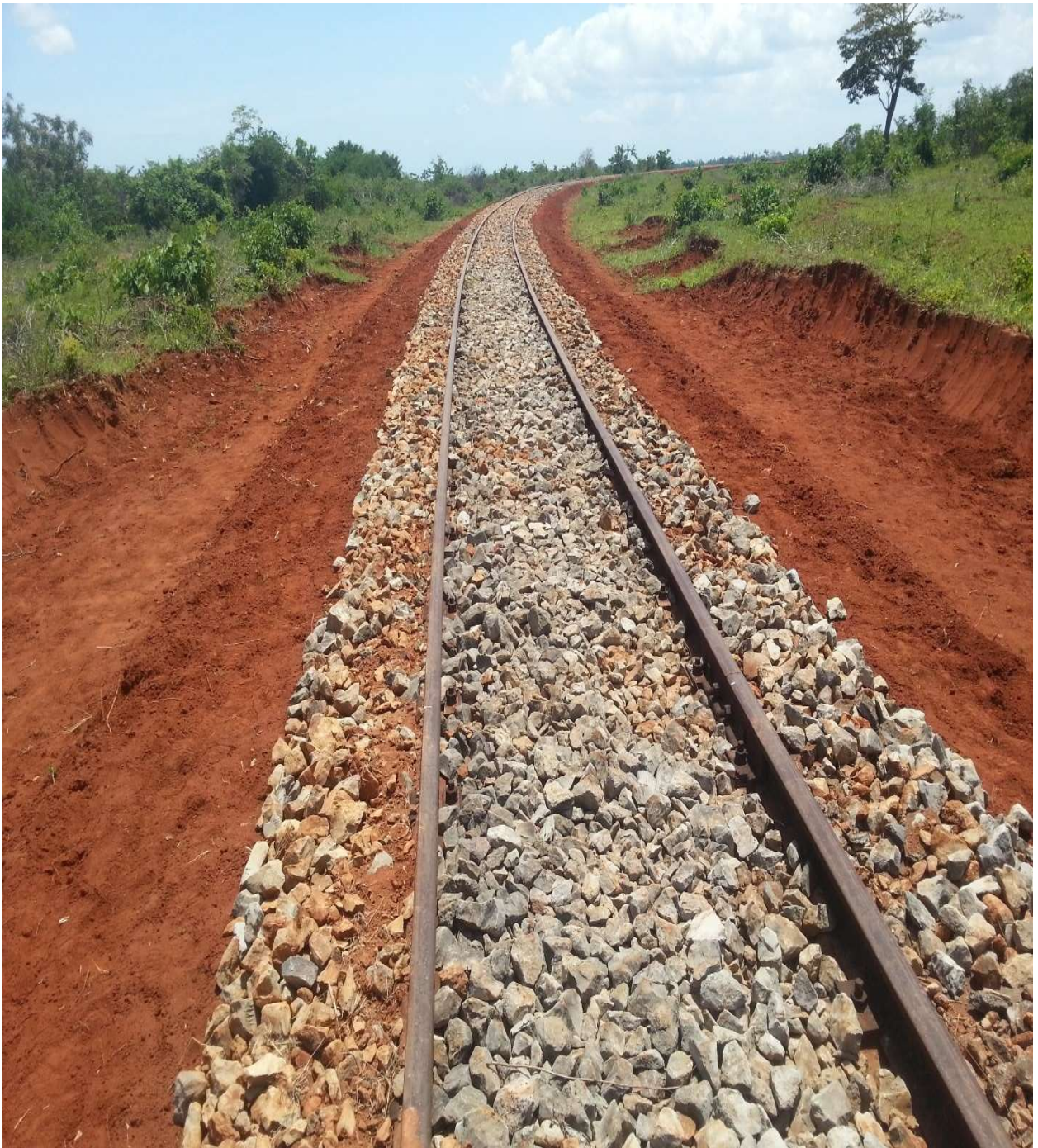
Track maintenance rebuilding of embankment at Tanga Cement factory line
