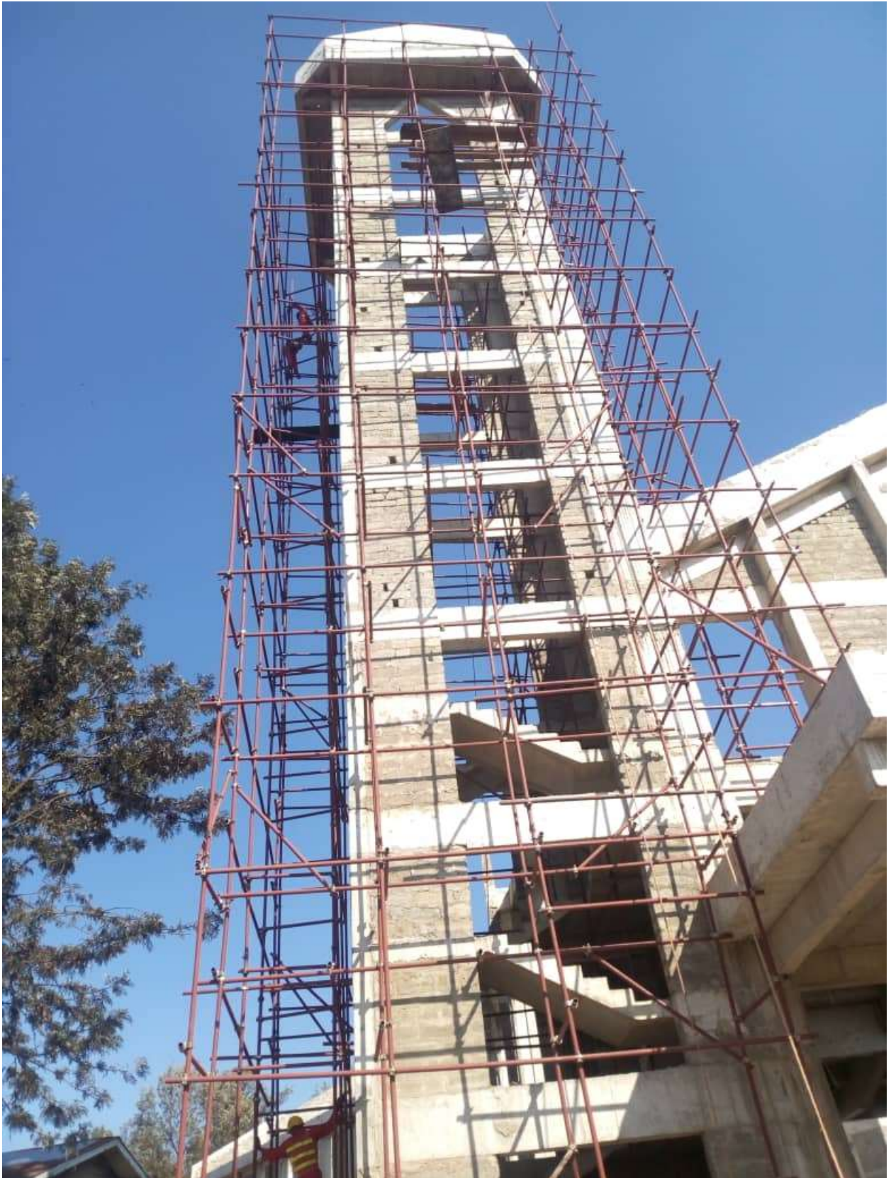
Scaffold erection for rear spire at St Theresa Cathedral, Arusha
