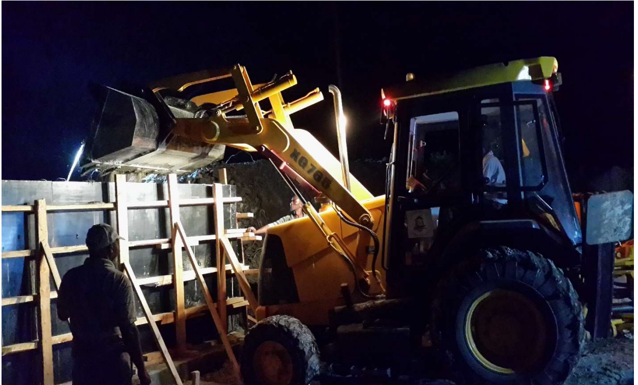
Backfill to cross drainage works along Ruvu - Mruazi railway Line
