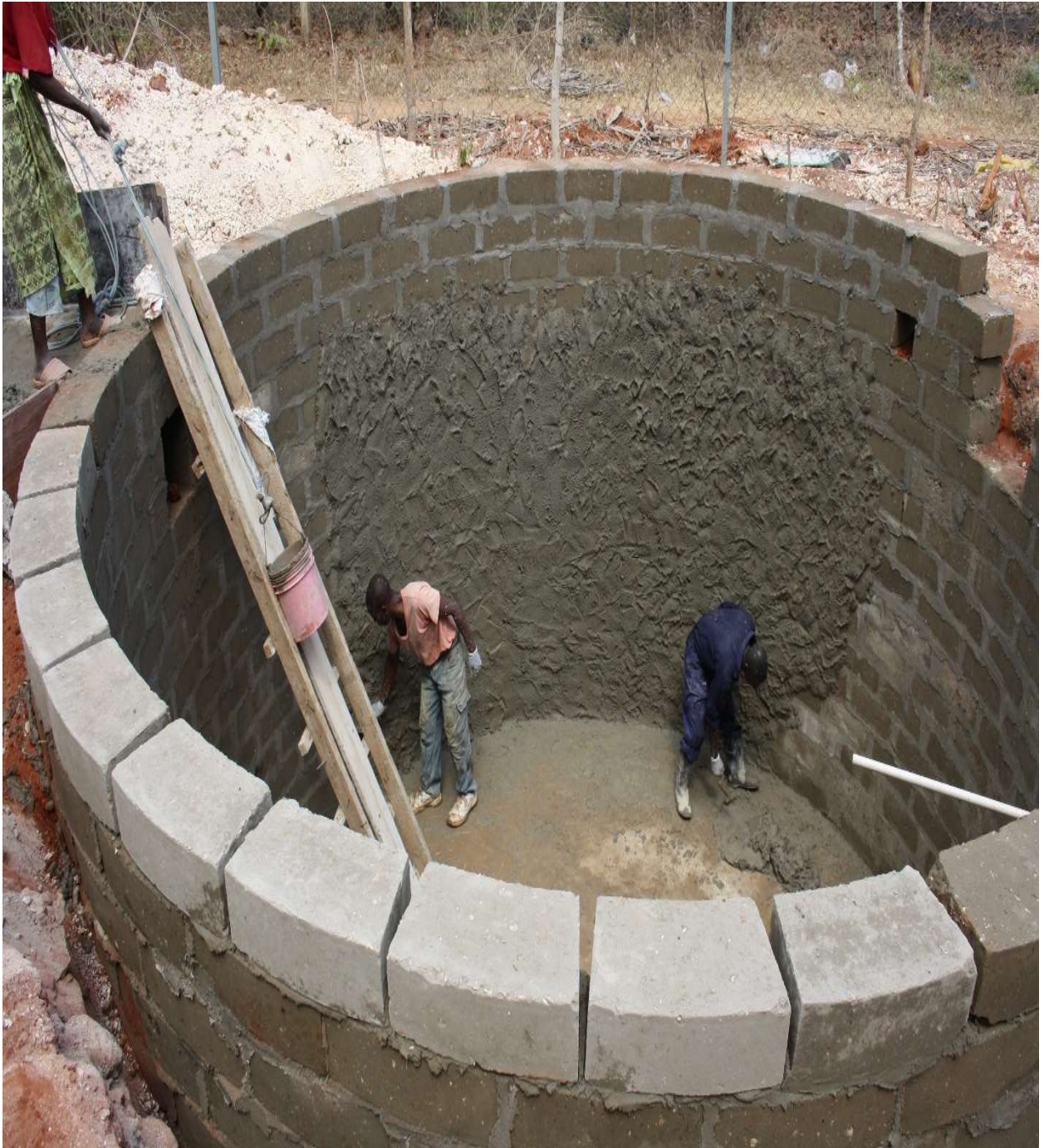
Construction of rainwater harvesting storage tank at Stella Maris University hostel, Mtwara
