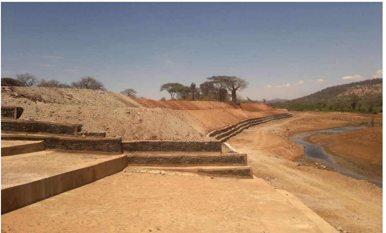
River training on the Kaliua to Mpanda Railway Line
