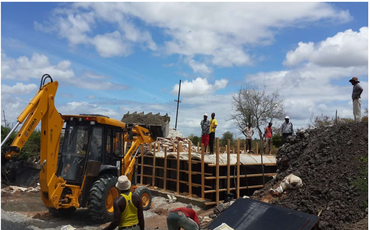
Emergency Reconstruction of collapsed culverts to restore line operations, Ruvu-mruazi link line
