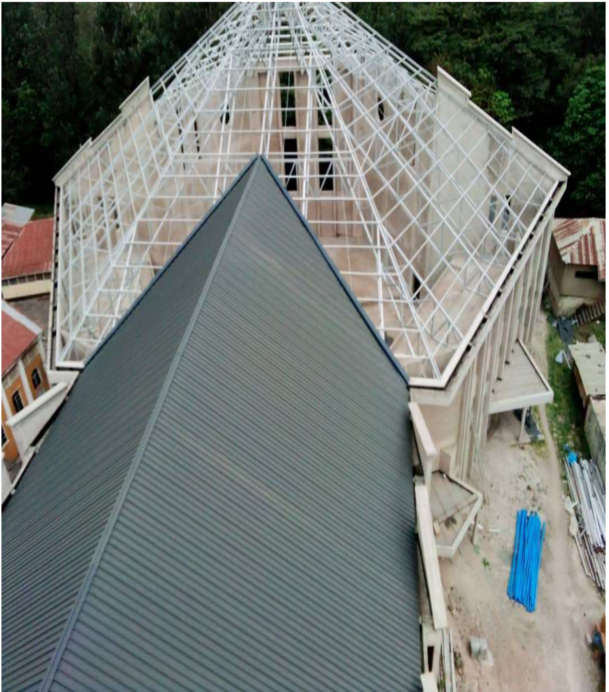
Roof covering in progress at St Theresa Cathedral, Arusha
