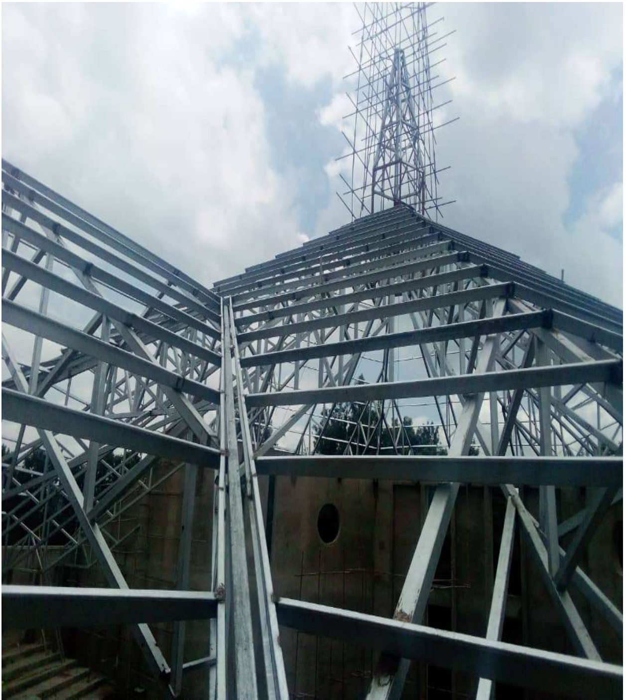
Altar spire erection at St Theresa Cathedral, Arusha
