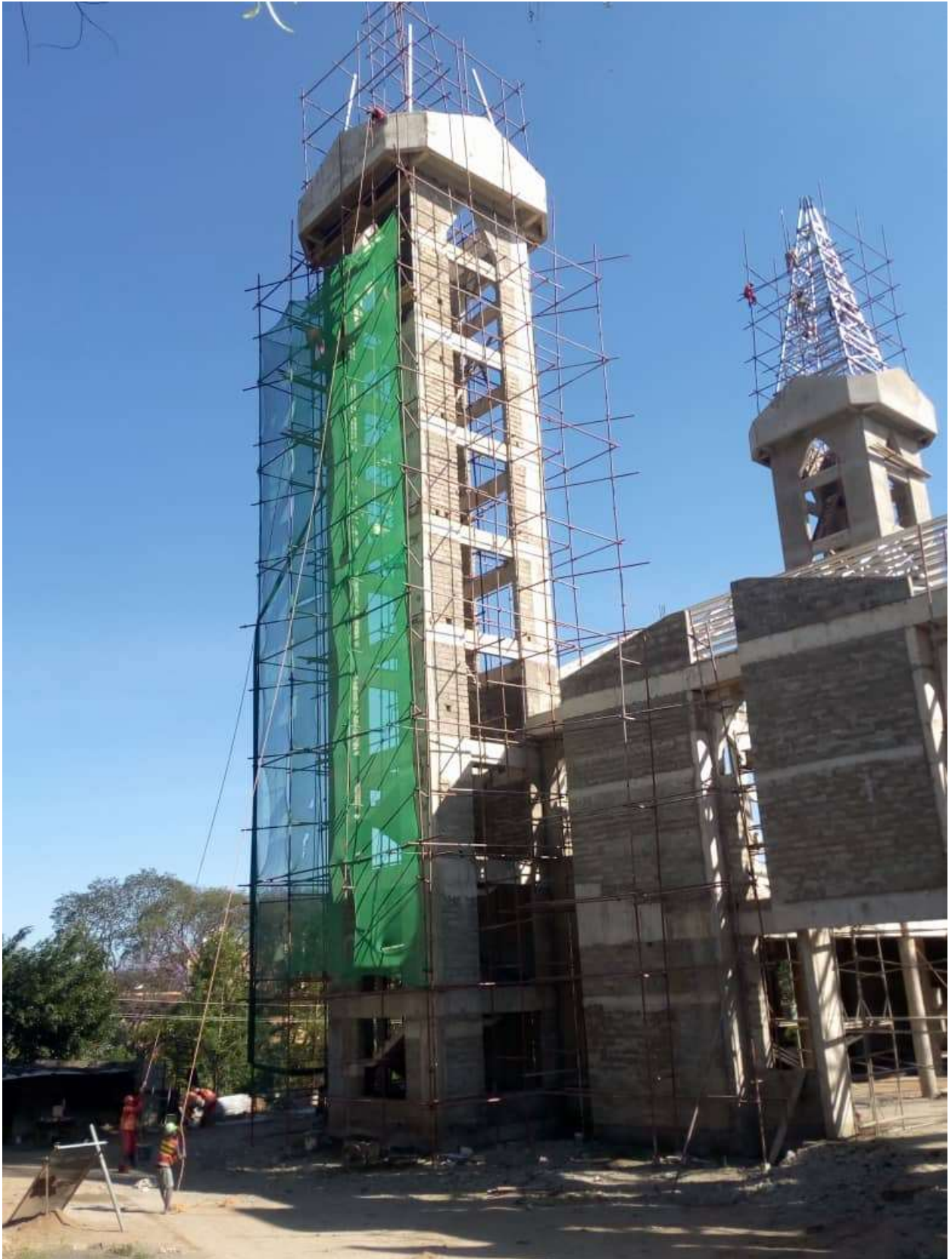
Rear spire truss fixing at St Theresa Cathedral, Arusha
