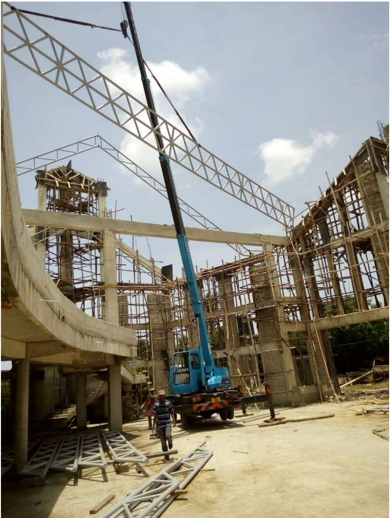
Truss erection and fixing at St Agustino parish Salasala, Dar es Salaam
