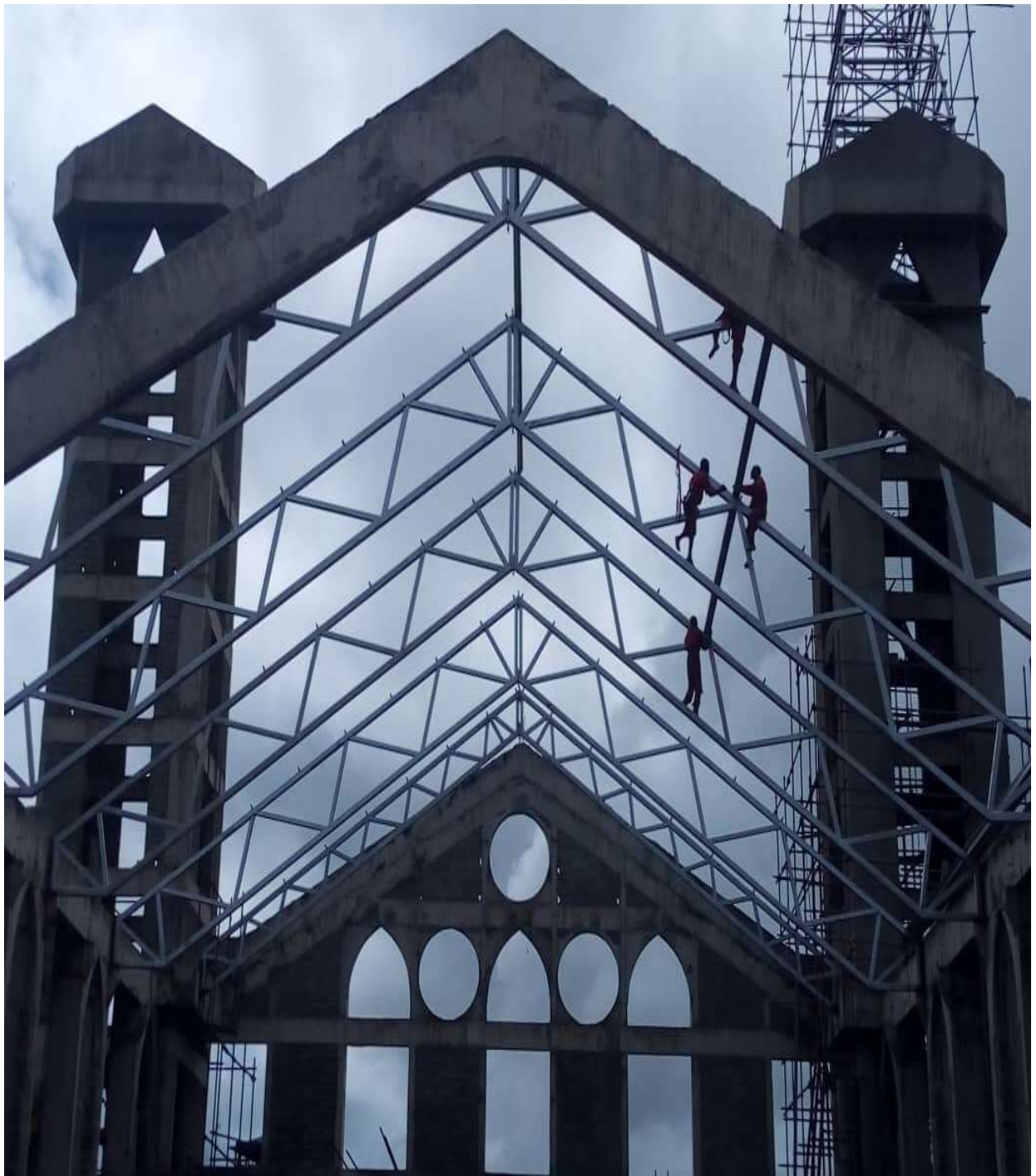
Truss erection and fixing at St Theresa Cathedral, Arusha
