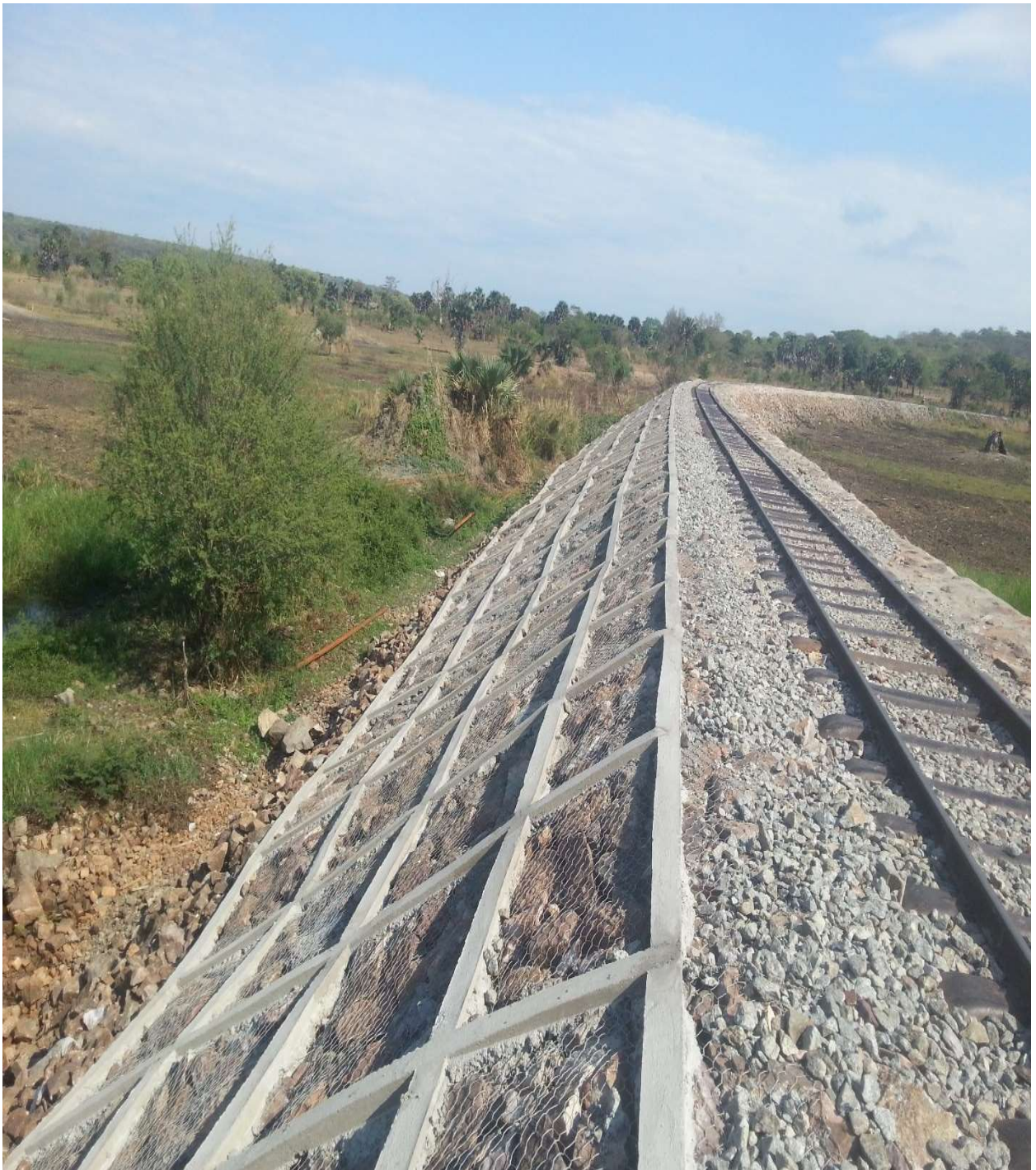
Protection of Ugalla river course way by boulders against slippage using gabion mattresses and concrete strips downstream
