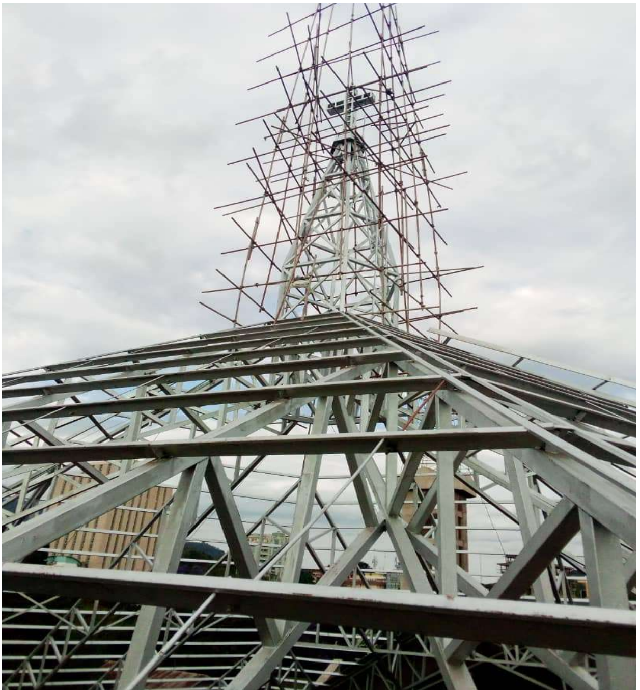
Galvanized cross fixing on St Theresa Cathedral altar spire, Arusha
